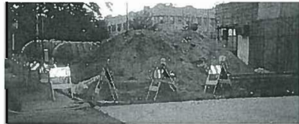
Underground storage tank upgrade
